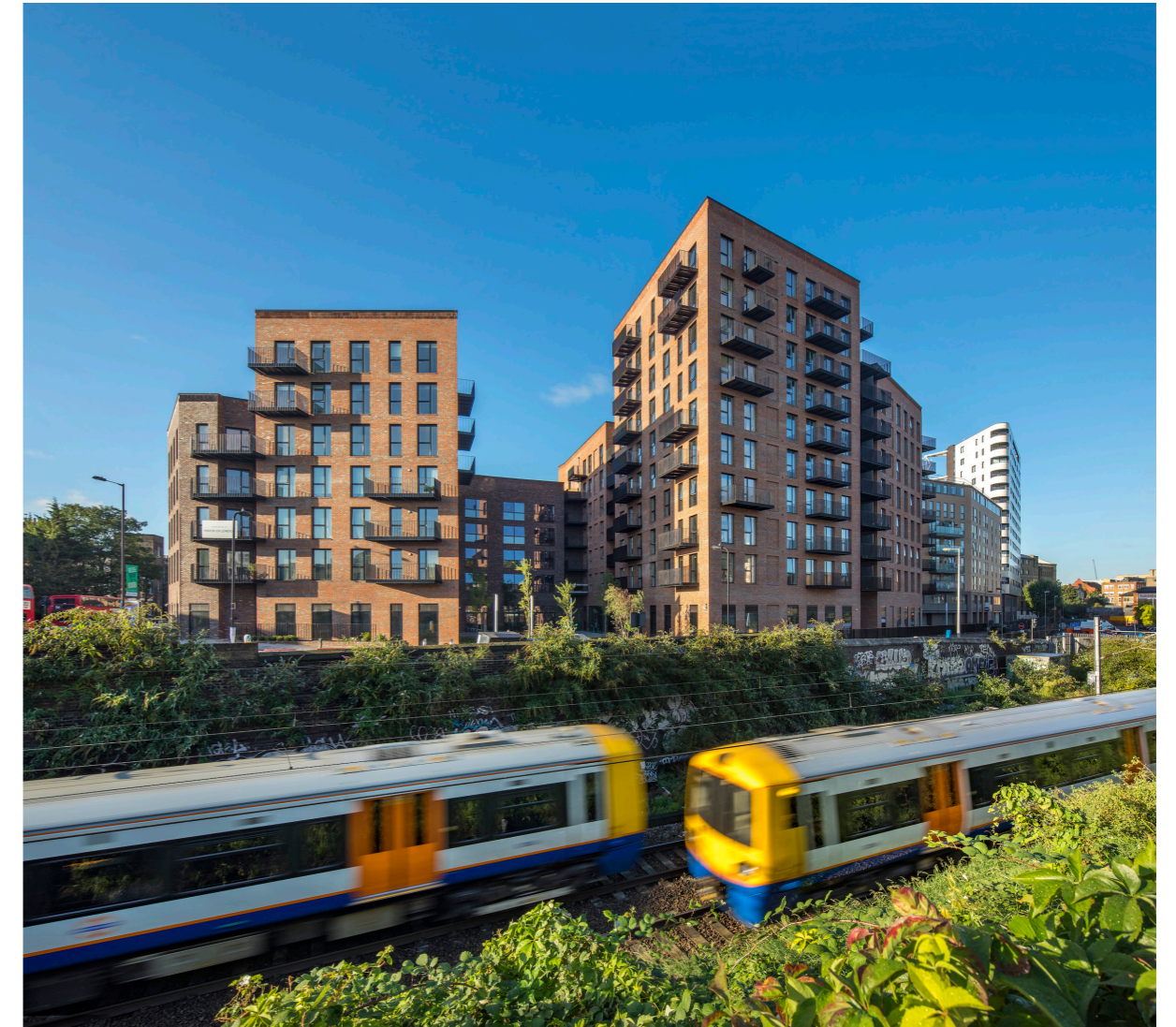
Bild 22: Dalston Lane, London. Waugh Thistleton Architects.
